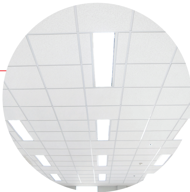
False ceiling elements and building components
